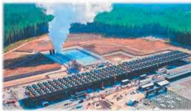
Fig.-1 Ngatamariki Geothermal Power Plant (Total reinjection of all fluids)
